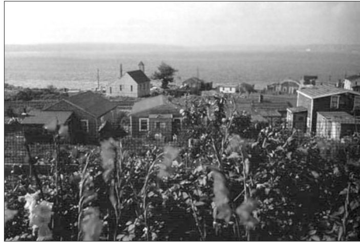
Before: Africville circa 1984; the community was denied basic sanitation and water services by the city of Halifax.
