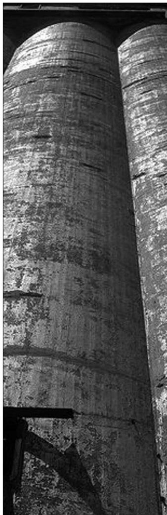
Cargill-owned grain elevators on Lake Erie. amerune
