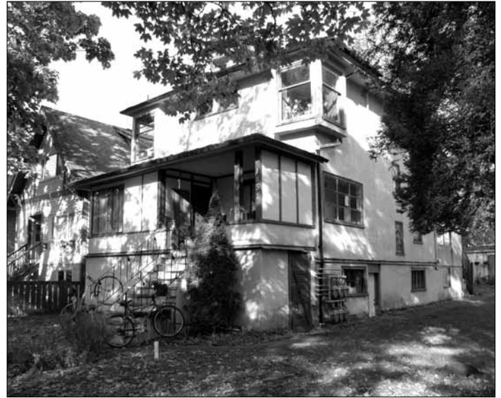
Tenants are being evicted from this Vancouver home despite the fact the owner does not have permits to demolish the house. Isaac Oommen
