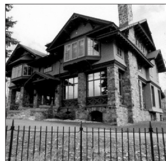
2002: Wilson House at Meech Lake, where the Ottawa Initiative took place.
